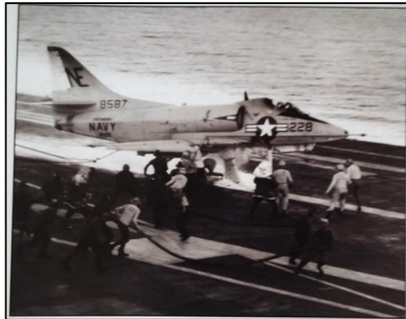
**Fig. 2** Lt. Ilg's A4 on Midway's flight deck showing the vertical stabilizer of the other A4 embedded in the underside of his plane (look directly below the intake). This photo was probably taken from Pri-Fly.
